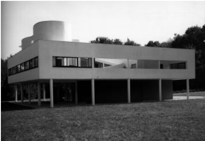
Figure 21: Le Corbusier, Villa Savoye (Photo: Ralph Liebermann).
