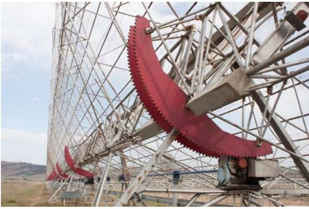
**Figure 3.** An overall image of the East-West arm of the Molonglo radio telescope showing the length and complexity of the metal structure and the motors and gearing systems required to make it move. Image: Wain, 2018.
