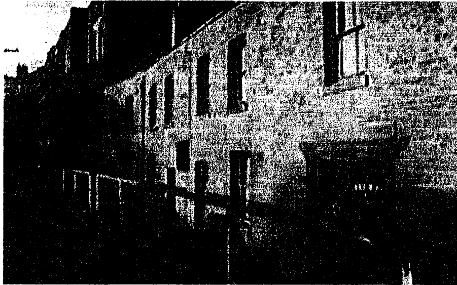
Illustration 18: The Susannah Place Museum, 58-64 Gloucester Street (Photograph © Richard Gange, HHT)
